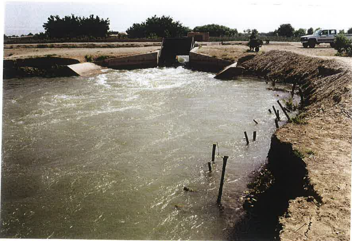
8. S-10.7 lateral intake gate off the Shamalan Canal with eroded wings and left bank service road. Note farmer placed sticks in an attempt at erosion control. The erosion resulted from years of no maintenance and the increase of water through the system. 24 April 2000
