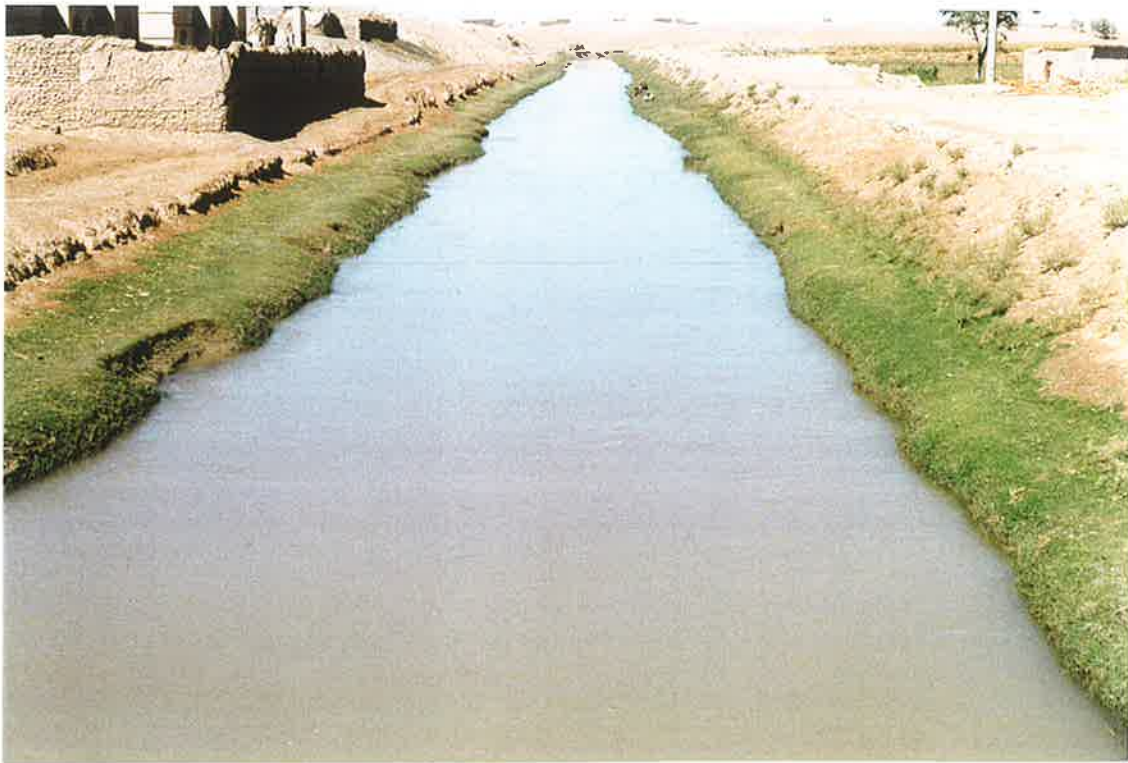
11. Silted banks of S-10,7 lateral at the Lashkar Gah to Marja road. The green grass is on silt to be removed, Note the compound wall built on the service road (top left). 10 Oct 97
