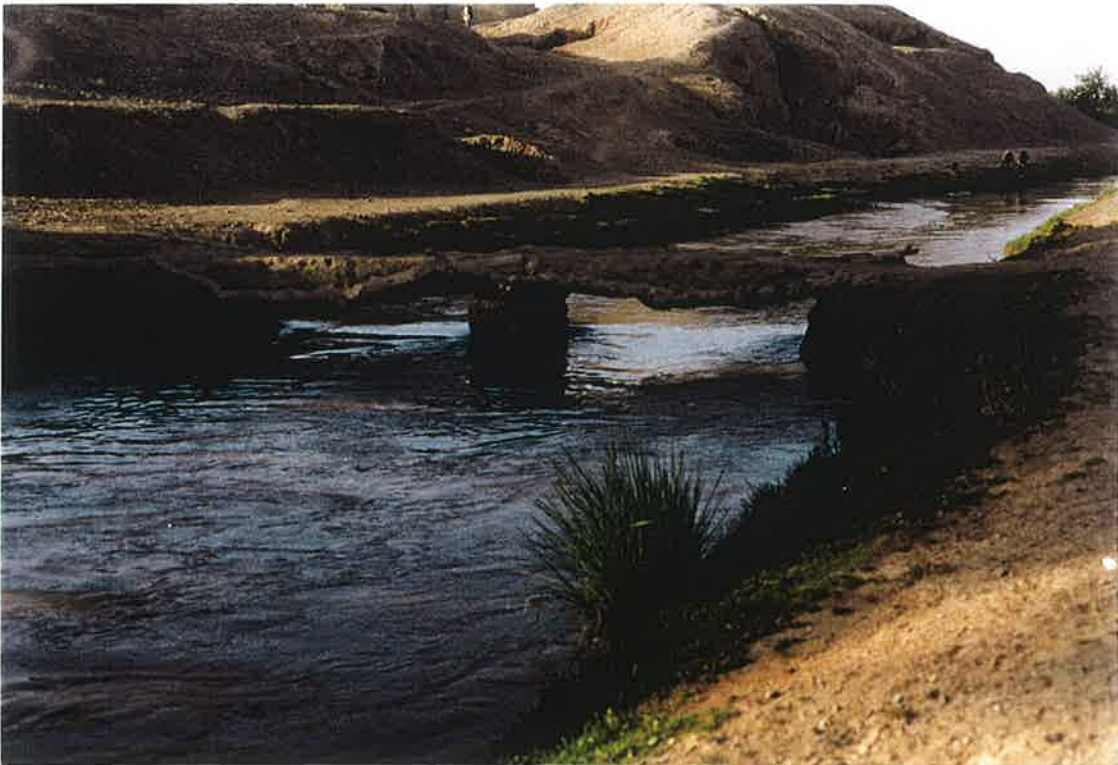
10. Farmer constructed bridge at \pm Km. 4 on S-10.7 lateral that constricts water flow. 20 April 98.
