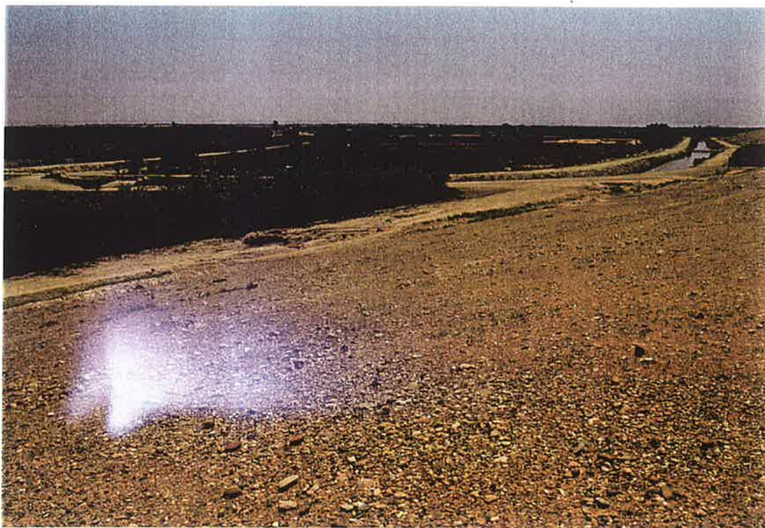
2. S-10.7 lateral at the Shamalan canal intake, Km. 0, on 20 April 1998. Note narrowing of channel by silt build-up.
