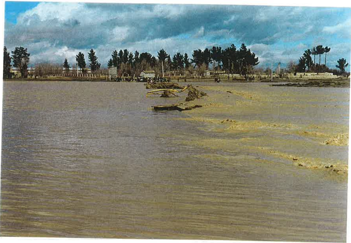
7 February 1999: Flood at Chan-I-Anjir footbridge. Note traffic jam at start of vehicle ford, top center. HAVA heavy equipment yard buildings are at top left, inside fenced area.
